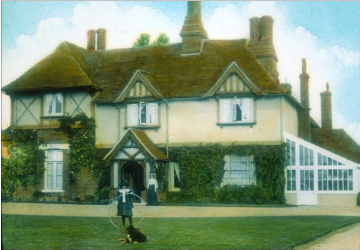
Fig 7: Davington Court around 1900 after 'renovation'.
